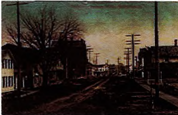
View north on Main Street, c. 1900
