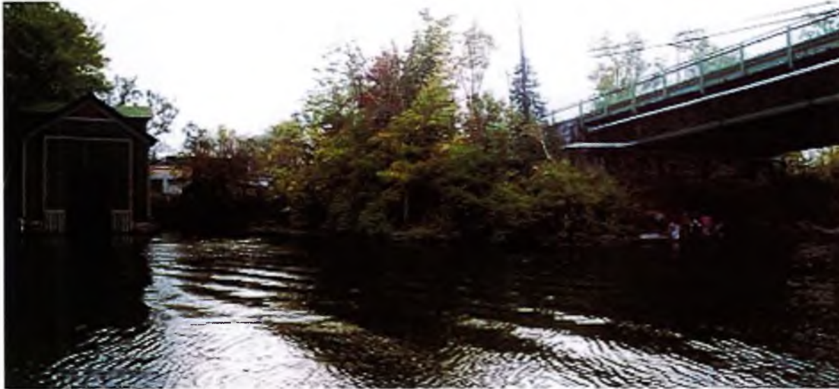
Existing view of Route 11 Bridge abutment
