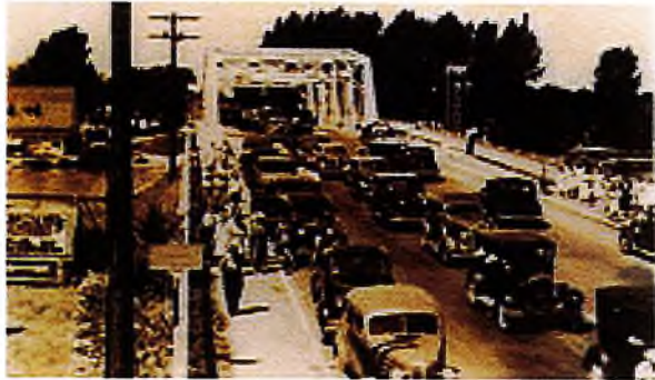
View north of the Brewerton Bridge, c. 1940
