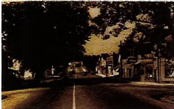
View north of Route 11, c. 1940
